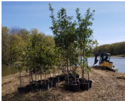
Pool 12 Forest Restoration MVR
