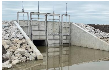
Clarence Cannon Water Control Structure MVS
