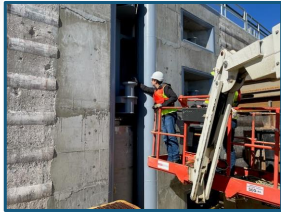
Lock 25 Phase 1 – Construction Complete
