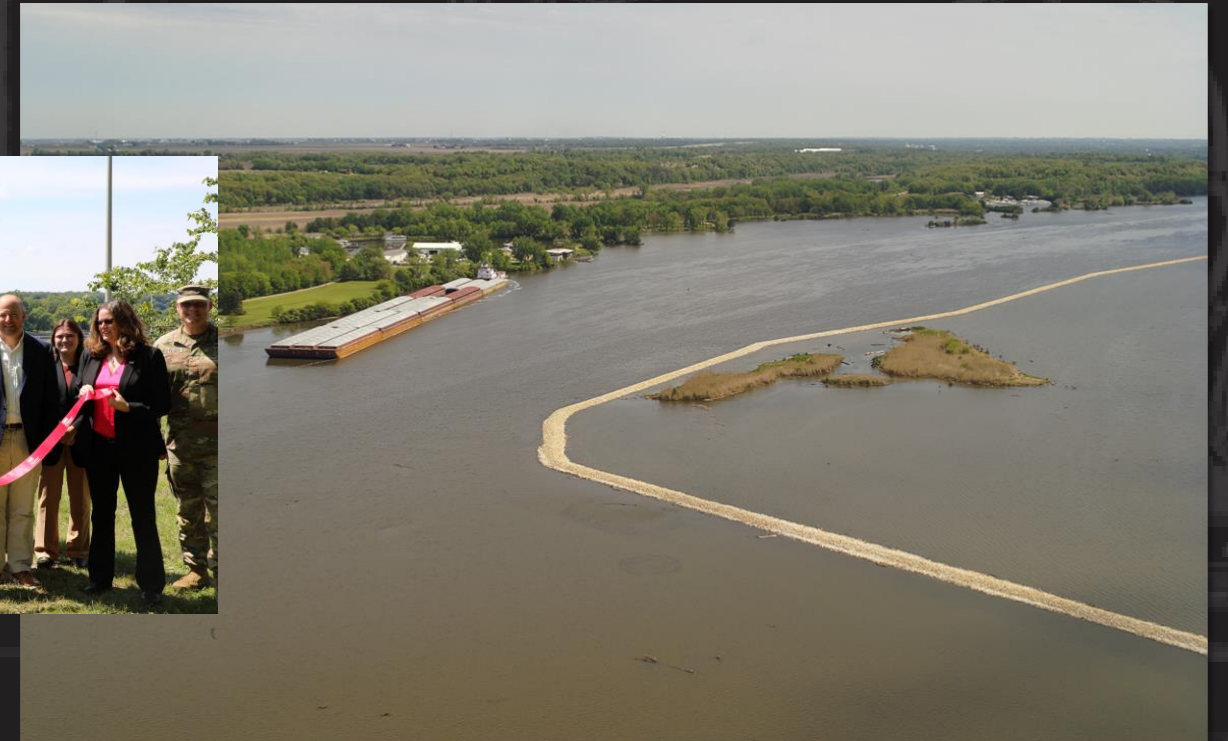
Starved Rock Habitat Rehabilitation - Project Complete
